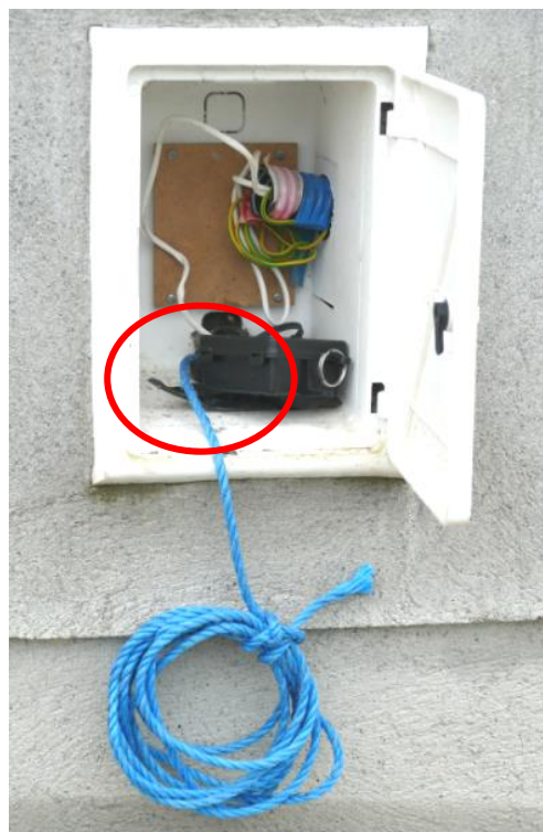
ETU at premises with draw rope installed.
